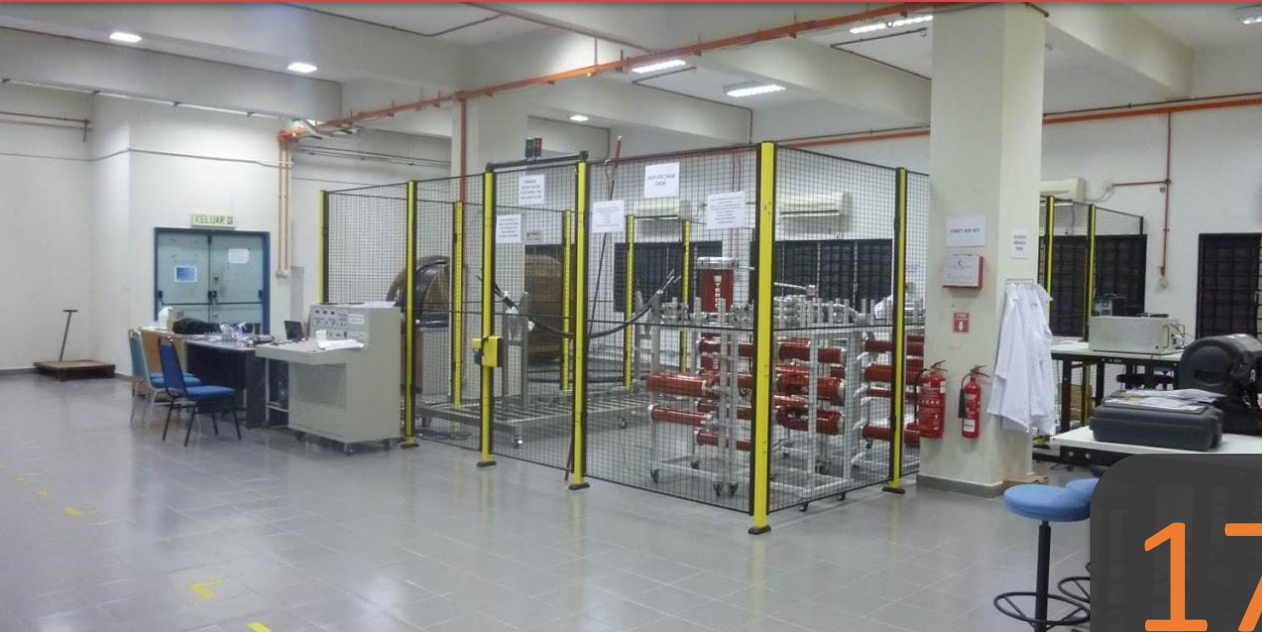
High Voltage Lab
